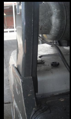
X – Unacceptable damage to overhead guard
